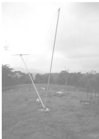
13m tower in 3/4 tilted position
