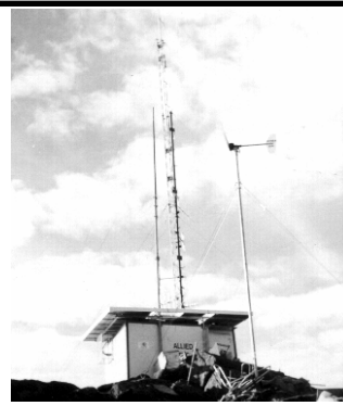
Professional Telecommunications Site Papua New Guinea - 14000ft.
